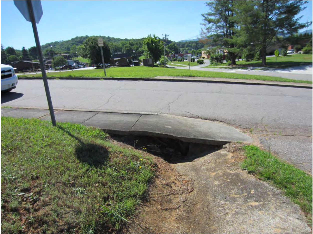
Photo showing the need for ADA-compliant curb ramps, handrail and marked crosswalk in front of stop bar for stop sign on Watauga St.
