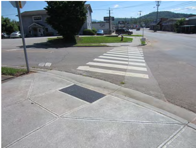
ADA-compliant Ramp with Detectable Domes
