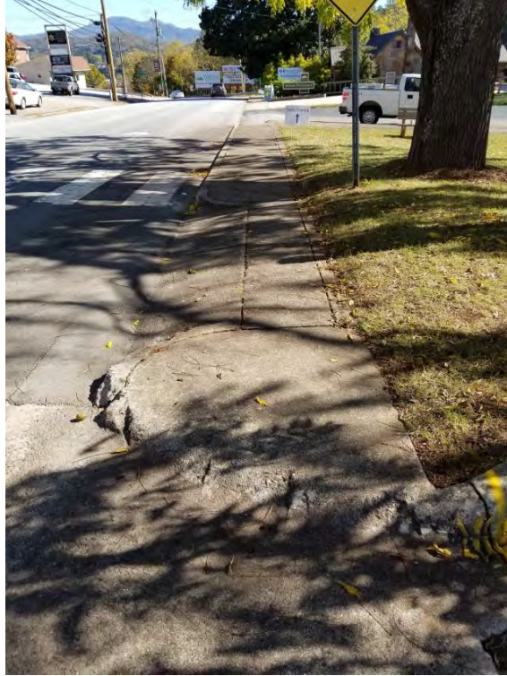
Cross Slope (Driveway Cuts)
