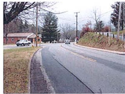
5. Facing Southwest on West Main Street
