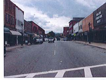
12. Facing Southwest on Main Street
