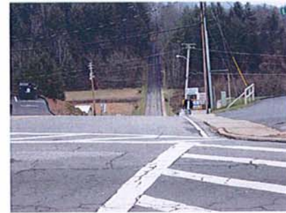
3. Facing South on Phillips Street
