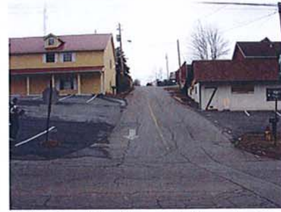
8. Facing North on Patton Ave.
