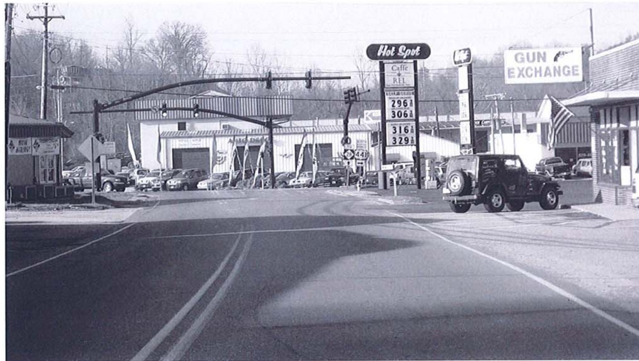
Existing Depot St. facing North
