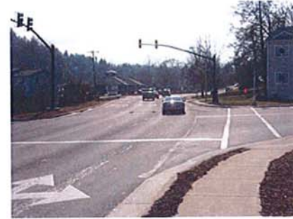
7. Facing Southwest on Main Street
