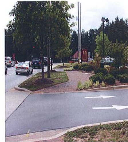
Parking Lot Improvements
