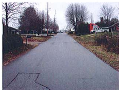
3. Facing North on Wilkie Street
