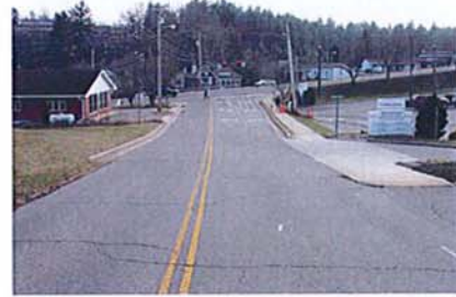
2. Facing Southeast on Riverview Street
