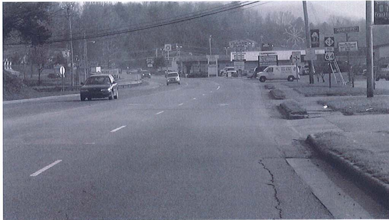
Existing Highlands Rd. facing South
