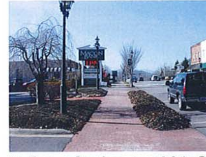
14. Facing Southwest on Main Street
