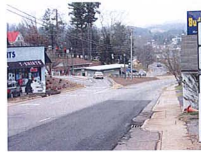
9. Facing Northeast on Patton Ave.
