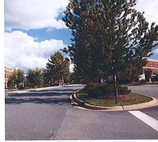
Parking Lot Improvements
